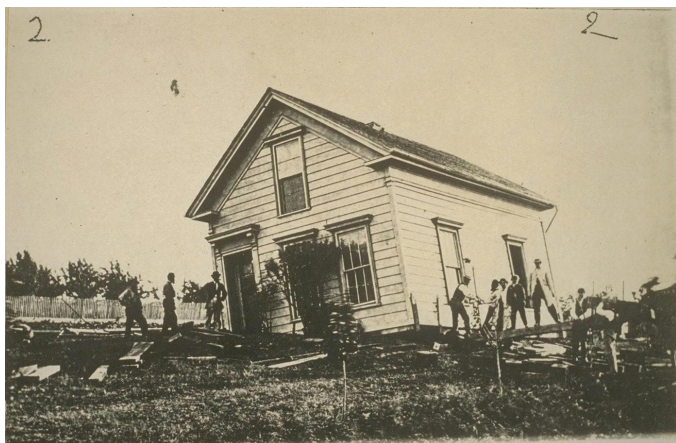
Fig. 4.21. Aftermath of an earthquake along the Hayward Fault, Hayward, CA (home of the author), 1868.
