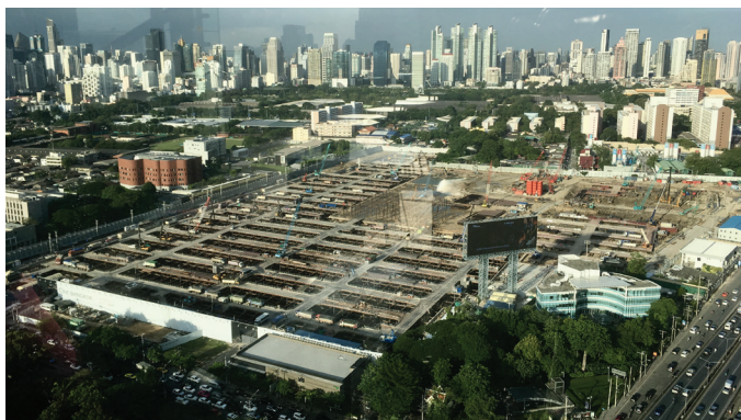
Figure 11.1. Preparation for the largest “Mat Foundation Pouring” in Southeast Asian history at Bangkok One, Bangkok, Thailand. In February 2020, 23,725 cubic meters of concrete was poured during a 33-hour period. Photo by Eli Elinoff.
