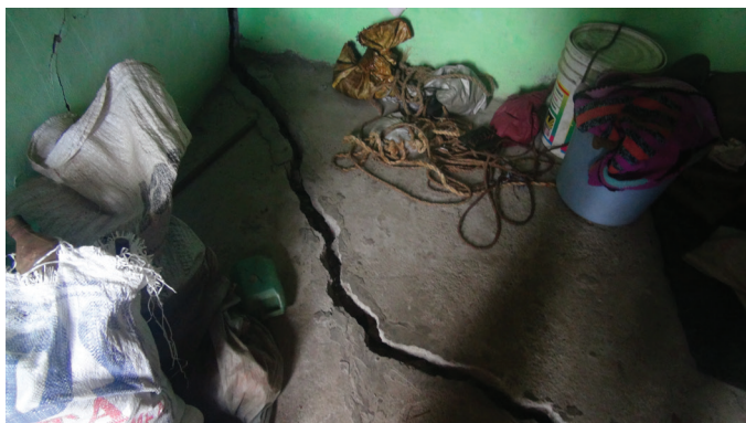
Figure 23.2. Cracked concrete interior, Indian Himalaya. Photo by the author.
