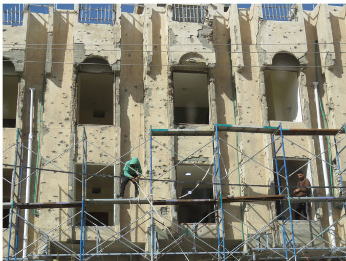
Figure 1.4. Bullet-riddled wall repair, Iraq. Photo credit: Debra Ellis.
