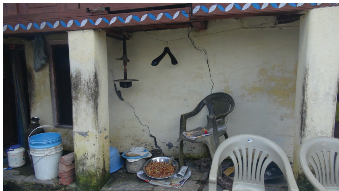
Figure 23.1. Concrete house with crack, Indian Himalaya. Photo by the author.
