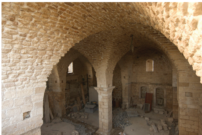
Figure 14.1. Interior of the house in the town of Shefa'amer in the Galilee after most of the concrete plastering was removed. Photo by the author, 2010.
