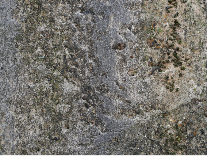
Figure 25.1. Bedford Way, London (July 2021). An urban microbiome has formed across the surface of the concrete with clear signs of biodeterioration caused by organic acids secreted by microorganisms. Photo by the author.
