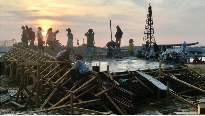
Figure 1.1. Construction workers pour and smooth a concrete pier in Hpa An, Myanmar. Photo credit: Eli Elinoff.
