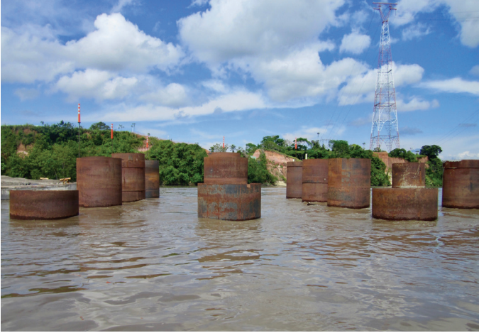
Figure 6.2. Piles to be filled with concrete, Puerto Berrío. Photo by the author.
