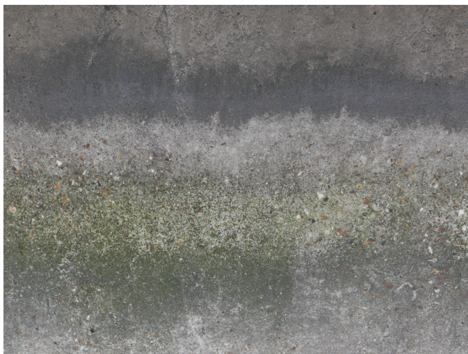
Figure 25.2. Bedford Way, London (July 2021). The greenish dark lower band of coloration is likely caused by algae. Photo by the author.
